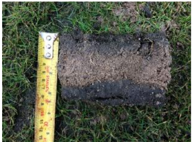
Figure 4: A shallow sand layer is apparent above the constructed profile and grass coverage is weak on the surface, with limited root penetration.
