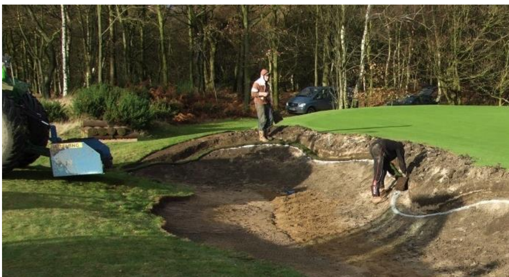
Installation of revetted turf lip on prepared shelf
