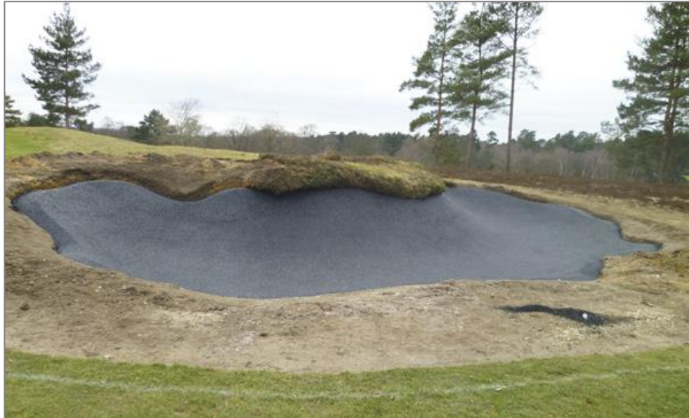
Bunker blinder installation at The Berkshire
